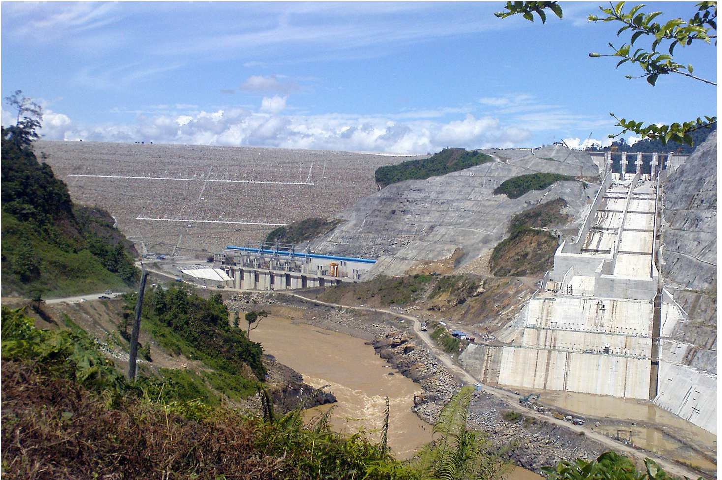
THE BAKUN DAM in Malaysia started operating in 2011.
